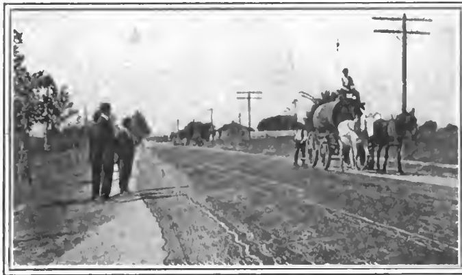
Oiling a straightaway in preparation for Savannah road races
